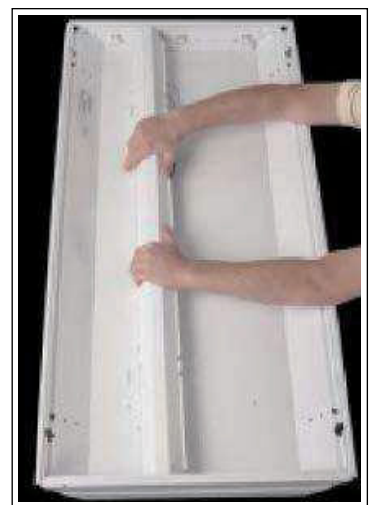
(c) Remove ballast cover (lens removed)
