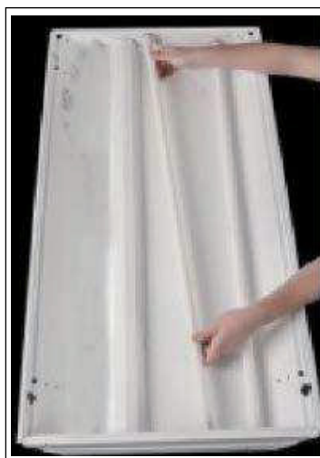
(b) Remove tube light source(s)
